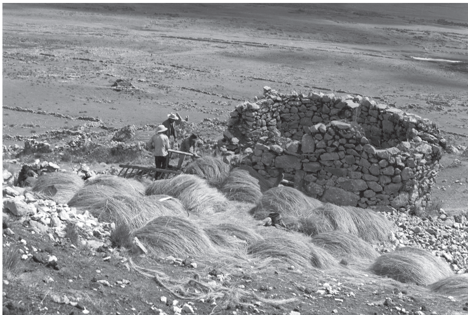
Figure 13. Workers assembling stacks of straw to reconstruct a roof for the “ Mama Qollqa ,” Huánuco Pampa. John V. Murra Archive; courtesy of the Division of Anthropology, American Museum of Natural History, New York.
